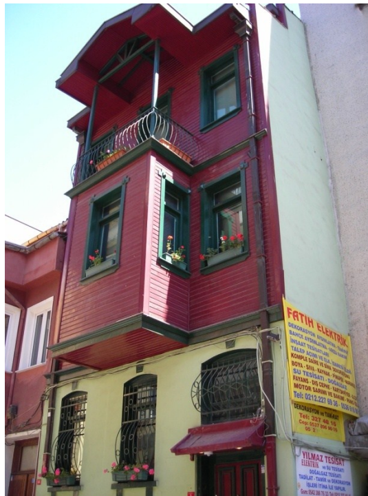
Fig. 3. A repaired house of native inhabitant (a) and (b) a “restored” house on the very same street, İstanbul
