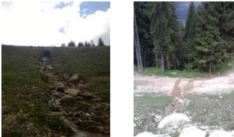
Fig. 7. and 8. Unsolved sewerage infrastructure in the Ski center Vlašić
