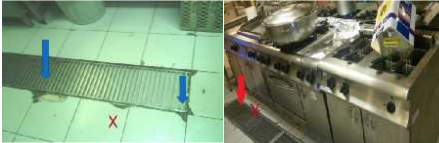
Fig. 1. (Continuation) Kitchen floor, walls and ceiling
