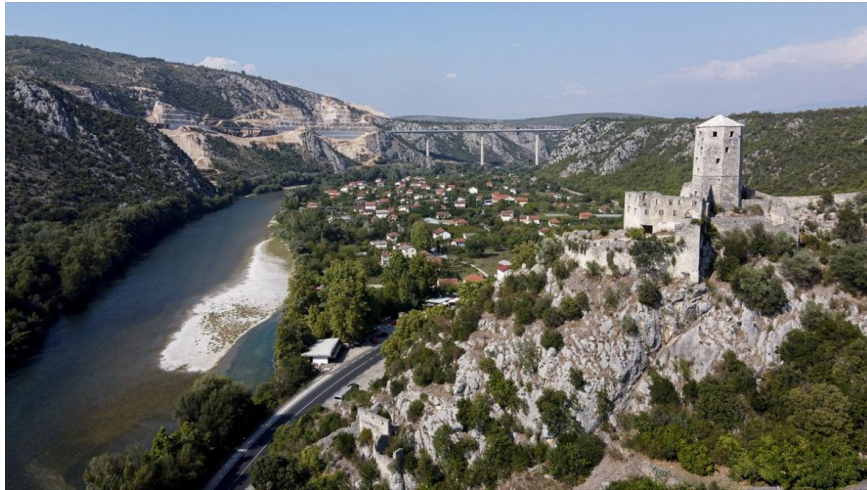
Fig. 3. Hercegovina bridge near Počitelj
